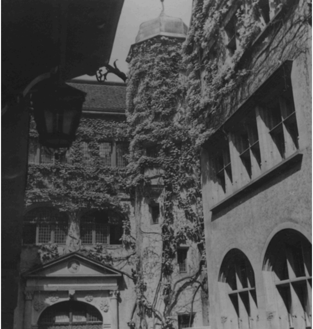
Figure 8: Freiburg City Hall
